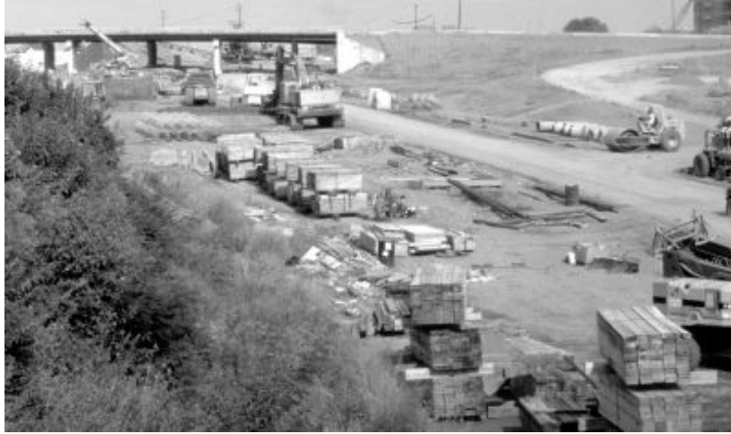
Figure 12. Example of Increased Available Workspace of a Full Road Closure (93)
